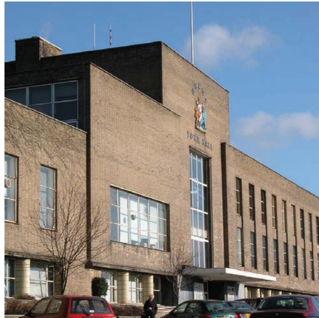
Picture 4.7 Brent Town Hall (Grade II)
