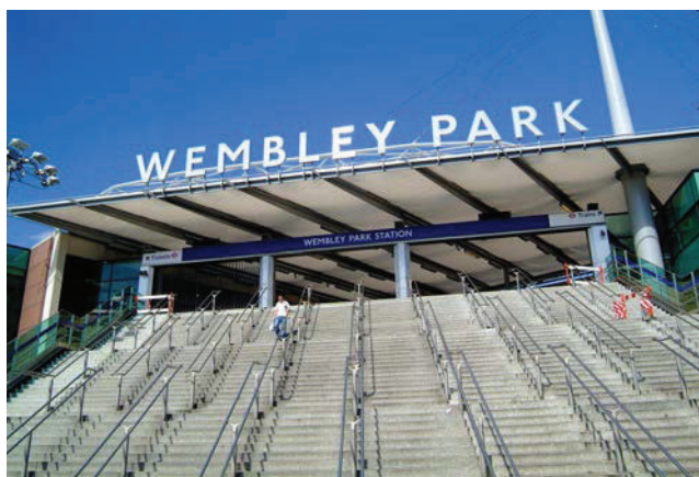
Picture 4.21 Wembley Park Station
