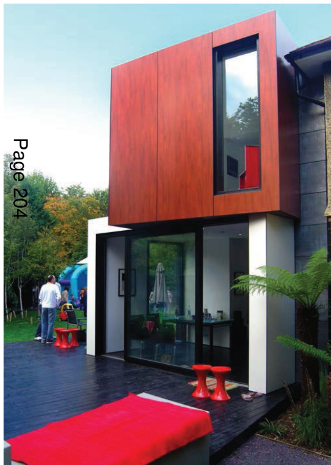
Picture 4.42 A well detailed contemporary home extension
