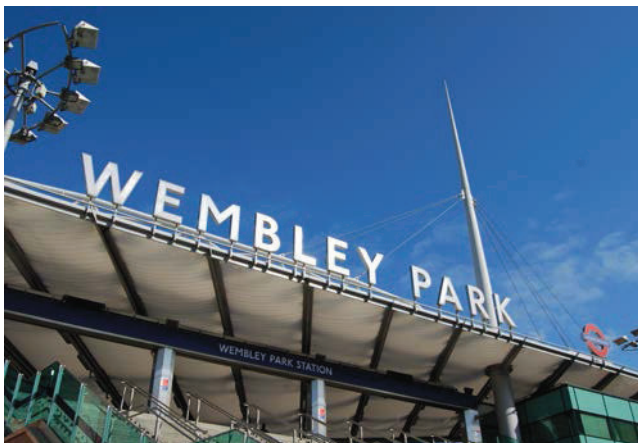
Picture 4.30 Wembley Park Station
